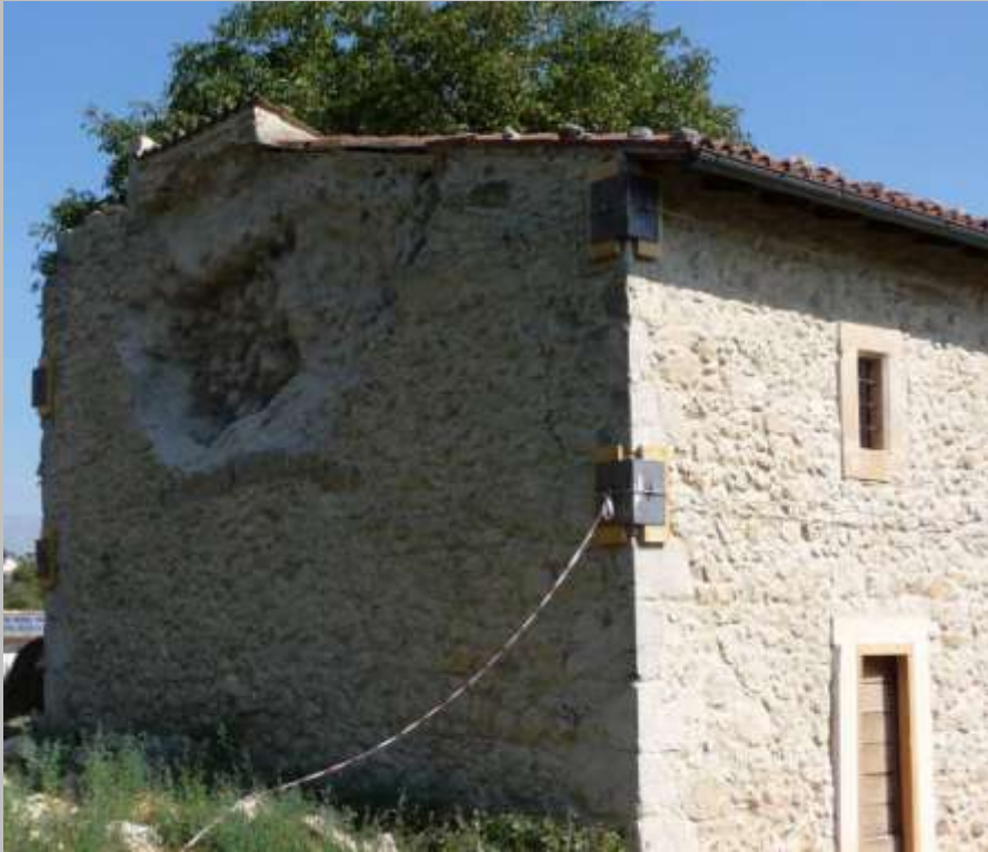
WALL STABILIZATION
